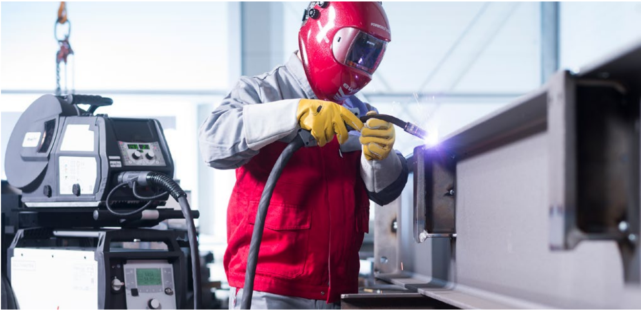
Figure 41: MAG welding in steel construction
