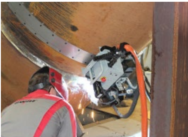
Figure 37: Fully mechanised GMAW orbital welding
