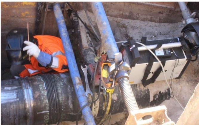
butt joint, both the valve side (-4 mT) and the pipe section (-12 to -18 mT) needed to be compensated at the second weld joint, likely due to the drifting of the magnetic field upon completing the first weld. This time, six coils were
